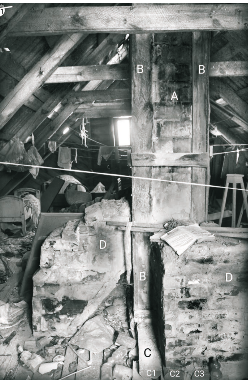
Fig. 11. The attic with the longest smoke flue (C) exposed; photos by the authors, 2018
