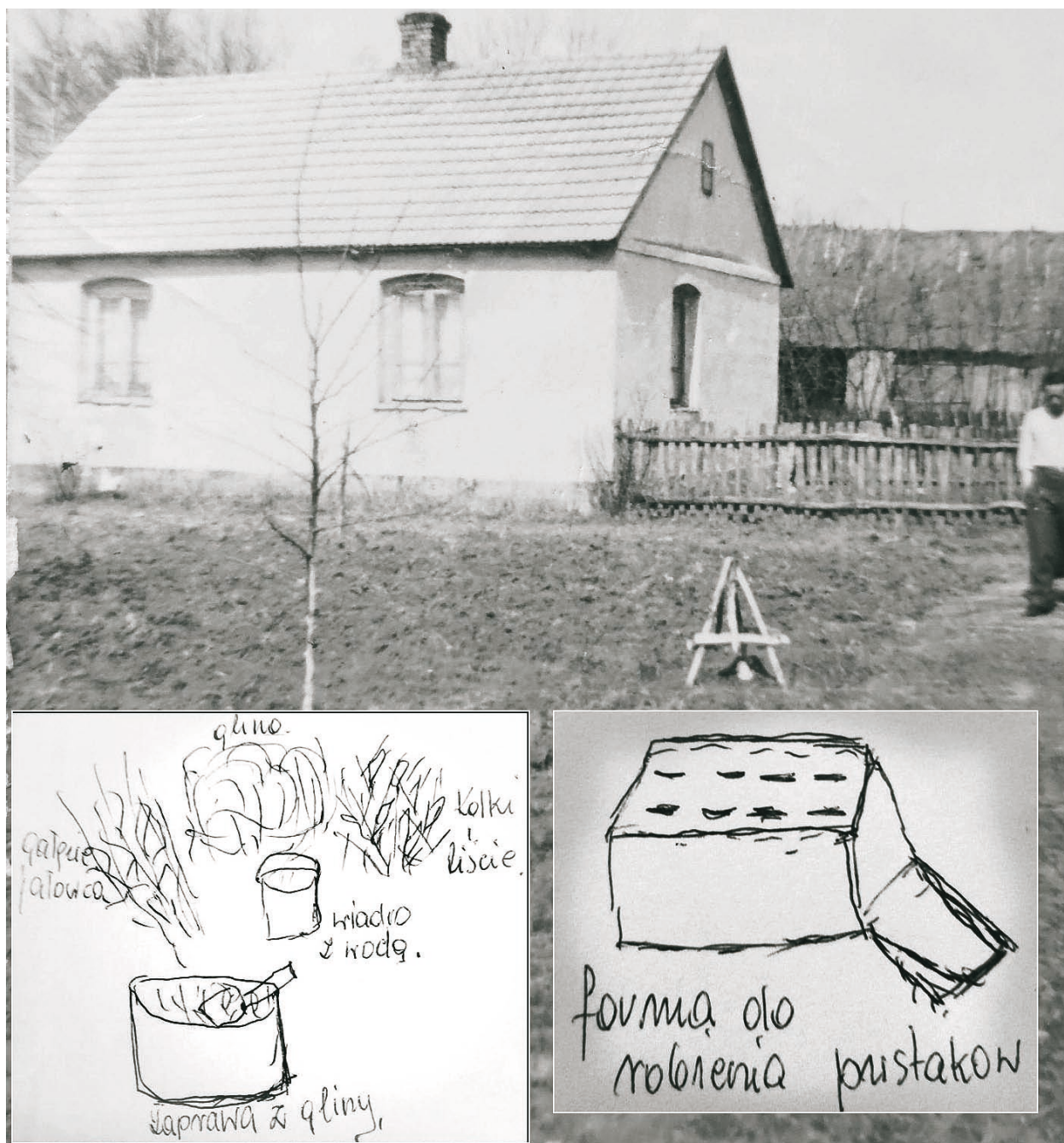
Fig. 3. An archival photograph of the earthen farmhouse; and the Interviewee's drawings of how building materials were made (cob for rammed walls, and a hollow brick mould) ; source: the family archive of Krystyna Kołakowska
