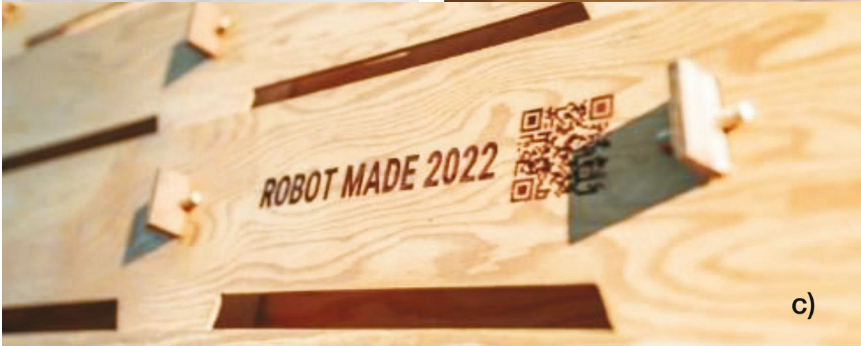
Fig. 8a–c. Mille-Feuille Pavilion, UBC, Vancouver, Canada, 2022, a) robotic CNC fabrication of plywood strips, b) wedging of joints, c) wedged mortise and tenon joint; source: O. Herwig 2023.
