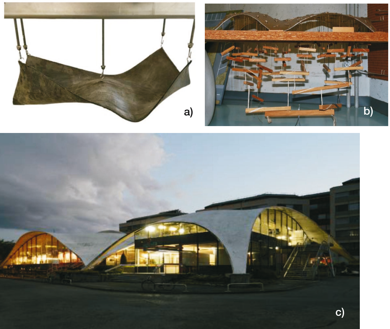
Fig. 3a–c. Heinz Isler, Sicli SA Factory in Geneva, 1968–1969, a) elastic rubber model small-scale epoxy resin model, b) the model used for the evaluation of structural behavior of the Sicli SA Factory in Geneva, c) Sicli SA Factory in Geneva; source: J. Chilton (2011); C.C. Chuang, J. Chilton (2016)
