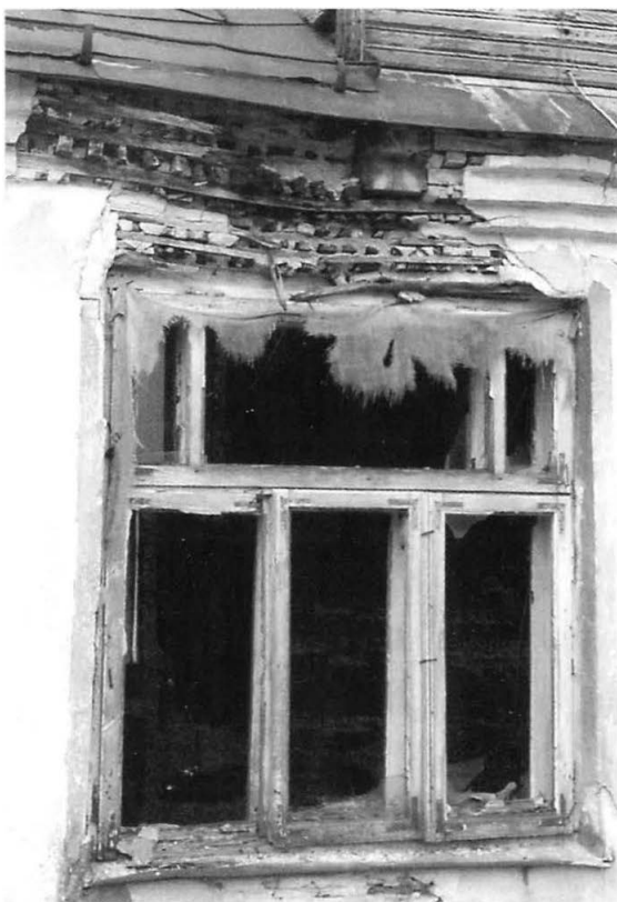
13. Okno i nadproże z gzymsem w domu z polan w Ploskach w gm. Bielsk Podlaski. Fot. Bogumiła Reczko, kwiecień 2002, Archiwum Zakładu Architektury i Planowania Wsi W.A. P.B. Window and lintel with a cornice in a house made of wooden billets in Ploski, commune of Bielsk Podlaski. Photo: Bogumiła Reczko, April 2002, Archive of the Faculty of Rural Architecture and Spatial Planning at the Department of Architecture at the Technical University of Białystok.
