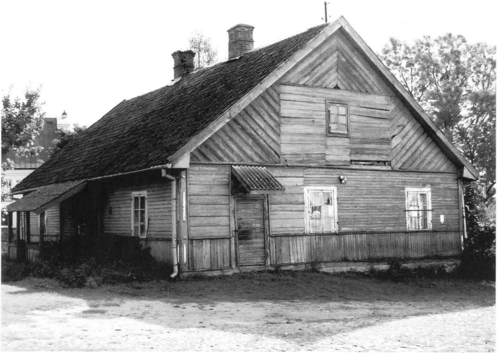
3. Widok ogólny plebanii z pn.-zach. Fot. J. Tołłoczko, 2005 r. General view of the vicarage from the north-west. Photo: J. Tołłoczko, 2005.
