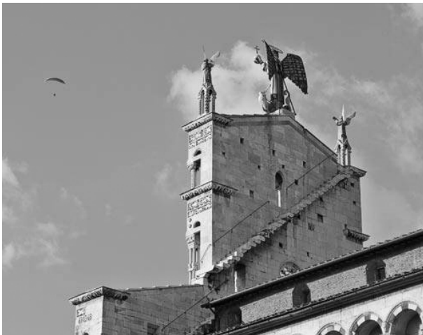
Fig. 7. View at the back of façade.
