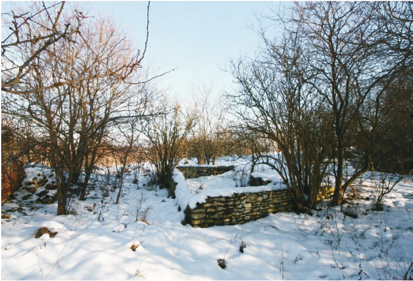
Fig. 9. Barn No. 4. The timber-constructed building has been completely destroyed. Remnants of the structure 2 a fragment of the stone foundation made of field limestone – have survived; source: photo by Andrzej Kos, February 2025.
