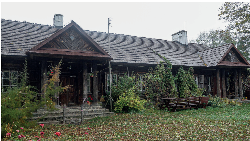
1 a i b. Oficyna dworska w Pobikrach. Dawny dwór rodziny Ciecierskich. Fot. N. Kamieńska, 2024 r. Manor annexe in Pobikry. The former manor house of the Ciecierski family. Photo by N. Kamieńska, 2024
