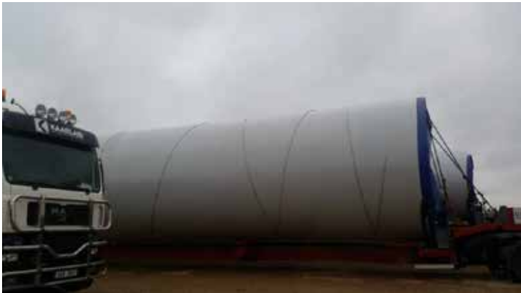
Fig. 3.12. Transportation and storage of wind turbine towers during the building of a wind turbine (farm) (Source: photos by T. J. Teleszewski (A) and K. Jasiūnas (B))
