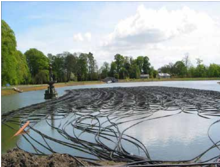
Fig. 5.31. An example of the air heat pump – external unit (Source: Smuczyńska, 2015)
