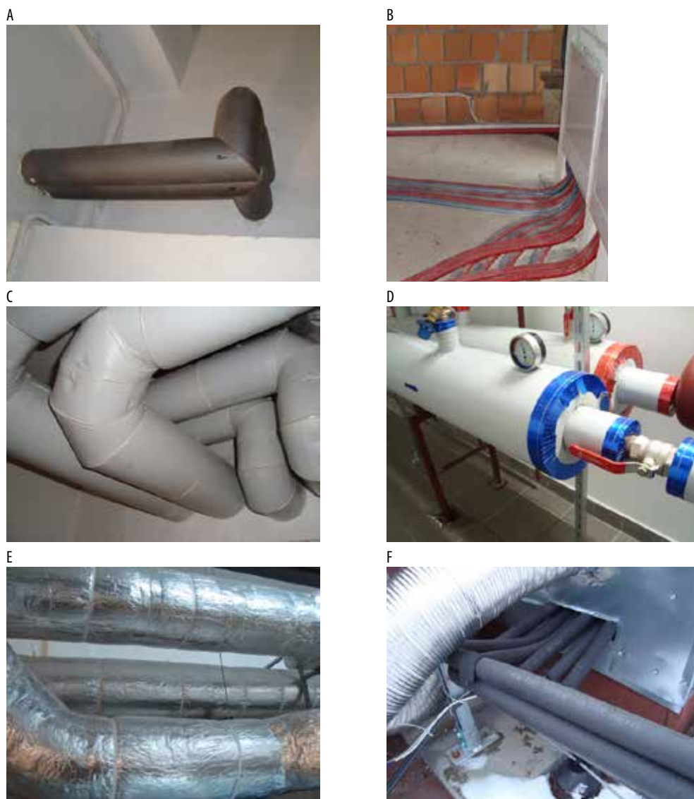
Fig. 7.17. Examples of insulation: A) foamed polyethylene without an outer coating, B) foamed polyethylene with an outer coating of polyethylene film, C-D) foamed polyurethane in a PVC housing, E) mineral wool with an aluminium foil coating, F) elastomer insulations (Source: A-CT.J. Teleszewski's private archive, D-E R. Bilinskienė's private archive)
