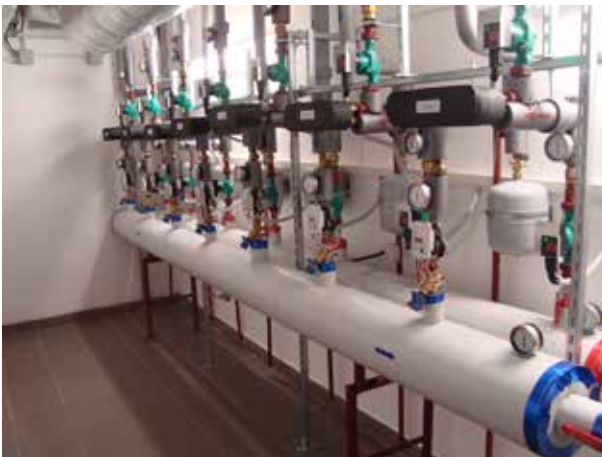
Fig. 7.19. Circulation pumps in a boiler room (Source: photos by T.J. Teleszewski)
