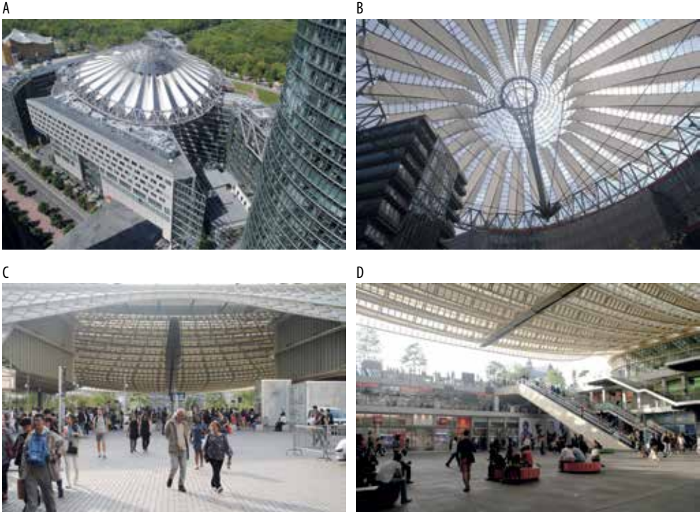
Fig. 1.20. Canopies on open public spaces. A, B) Sony Center (Berlin, Germany), C, D) Châtelet (Paris, France) (Source: photos by M. Kłopotowski)
