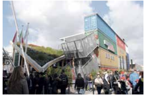
Fig. 1.8. The Monaco Pavilion from the World Exposition EXPO 2015 constructed of containers and other recycled materials (Milan, Italy) (Source: photos by M. Kłopotowski)
