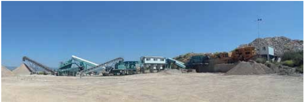
Fig. 3.21. Elements of a recycling plant. GECORSA, Córdoba, Spain (Source: J. R. Jimenez's private archive)
