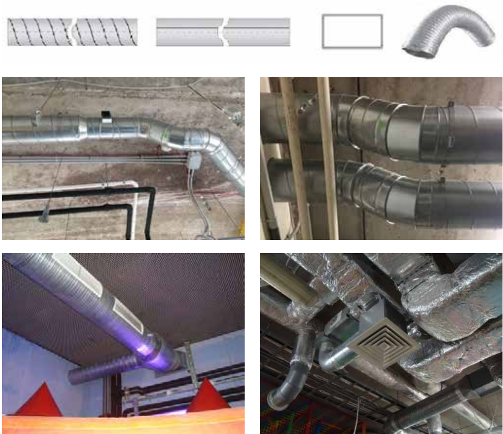
Fig. 8.6. Air duct types (Source: Bilinskienė, 2017; WEB-1,2; R. Bilinskienė's private archive; T.J. Teleszewski's private archive)
