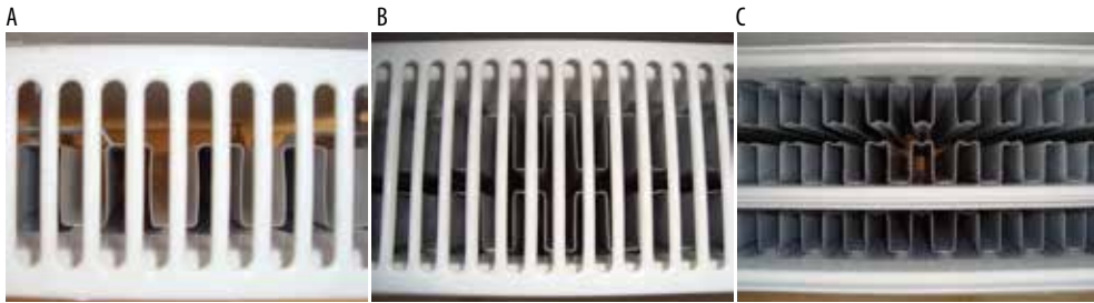
Fig. 7.6. View of the ribs in different types of flat heaters: A) 11, B) 22, C) 33 – radiator with the top cover removed (Source: T.J. Teleszewski's private archive)
