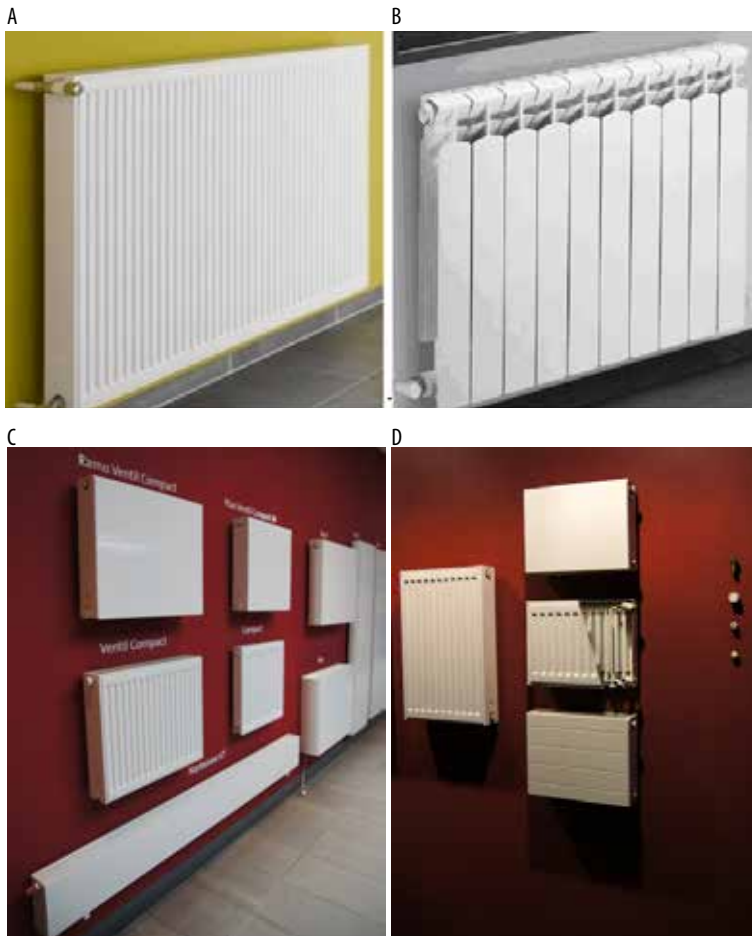
Fig. 7.5. Examples of heating devices. Radiators: A) panel radiator, B) column cast iron radiator C-D) different surfaces of panel radiators (Source: A) Bilinskiene at al., 2012, B) Bilinskiene, 2017, C) photo by D.A. Krawczyk, D) photo by E. Szatyłowicz)
