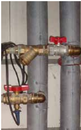
Fig. 7.4. The connection of the central heating installation: A) pipes distributed in a two-pipe loop B) the radiant heat manifolds (Source: T.J. Teleszewski's private archive)
