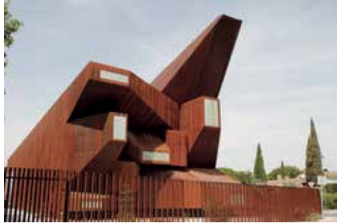
Fig. 1.32. Surprising form of the presbytery wall of Parroquia de Santa Mónica in Rivas Vaciamadrid near Madrid (Rivas Vaciamadrid, Spain) (Source: photos by M. Kłopotowski)
