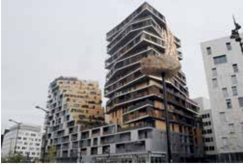
Fig. 2.22. Balconies surrounding a building completely change its spatial reception – Bâtiment Home in Paris XIII, France (2012-2015, architect Hamonic + Masson & Associés) (Source: photos by M. Kłopotowski)
