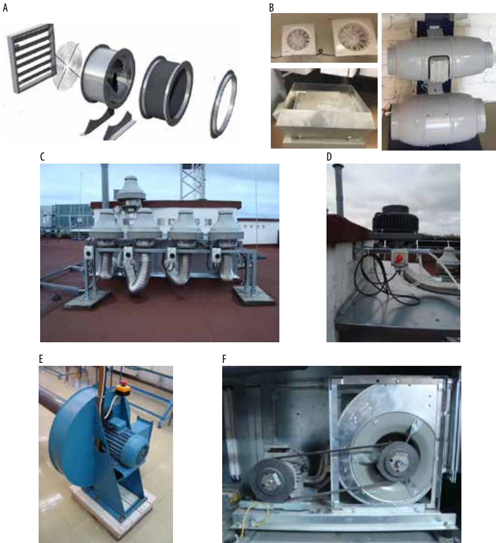
Fig. 8.7. Examples of fan constructions: A), B) an axial fan for installation in the ventilation duct and on the roof, C), D) axial fans installed on the roof, E) a centrifugal fan, F) a cross flow fan installed in the AHU unit (Source: Bilinskienė, 2017; WEB-1; R. Bilinskienė's private archive; photos by T.J. Teleszewski)
