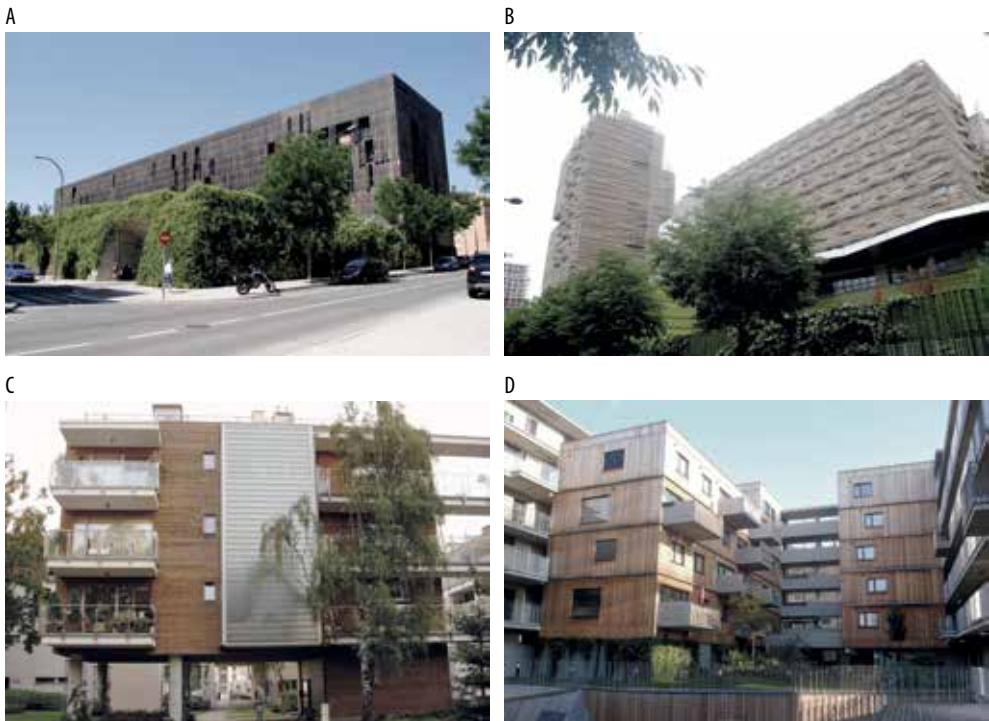
Fig. 2.33. Wood as a “new” pro-ecological building material. A) Moving shutters over the balconies around the Carabanchel Social Housing, Madrid, Spain (2007, architects Farshid Moussavi and Alejandro Zaera-Polo – Foreign Office Architects), B) Wooden openwork elevations School Group and Student Housing – Clichy –Batignolles, Paris, C) Wood-finished facades of the Allegretto Housing Complex in Eko Park in Warsaw, Poland (1999–2003, architects Stefan Kuryłowicz, Paweł Gumuła, Maria Saloni-Sadowska), D) Wood-finished facades and floors in Holzwohnbau in Seestadt Aspern, Vienna, Austria (2011–2015, architects Alfred Berger, Tiina Parkkinen – Architekten Berger + Parkkinen Ziviltechniker GmbH) (Source: photos by M. Kłopotowski)
