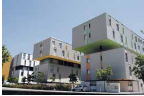
Fig. 2.23. Dividing a building into separate elements leads to the dynamics of the architectural form – Edificio Vallecas 5, Madrid, Spain (2006-2009, architects Luis Burriel Bielza, Pablo Fernandez Lewicki and Jose Antonio Tallon Iglesias – SOMOS Arquitectos) (Source: photos by M. Kłopotowski)
