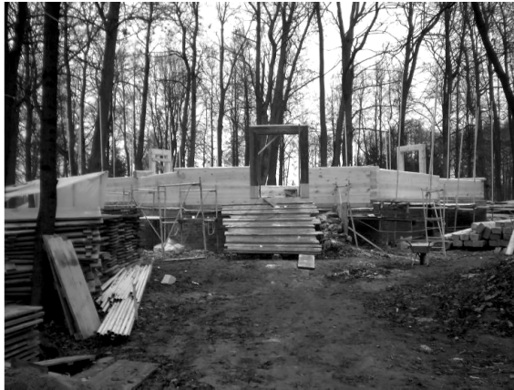
FIGURE 2.7. Construction work at the protection area
