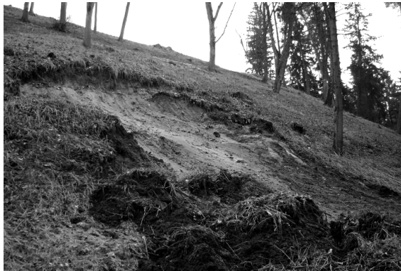
FIGURE 2.1. Erosion effected hillfort
