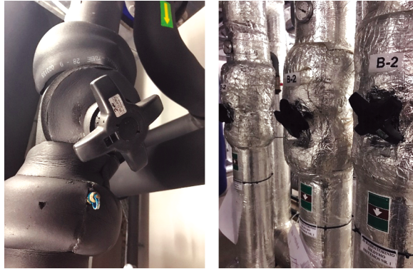
FIG. 2.14. Manual balancing valves (Source: Danfoss, 2022)
