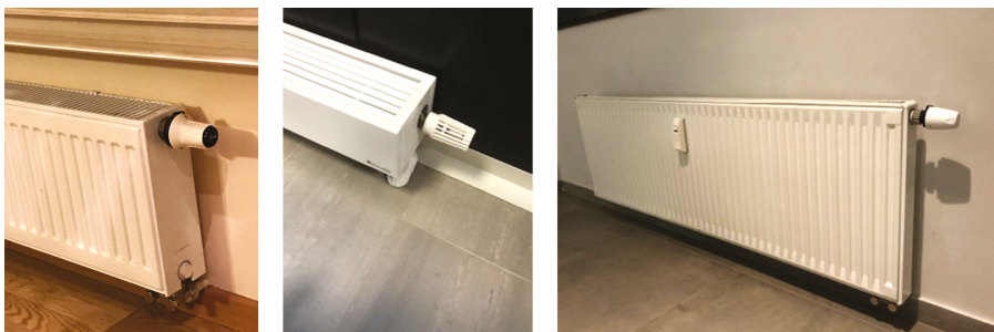
FIG. 2.19. Thermostatic valves installation examples (Source: photo by R. Bilinskiene)
