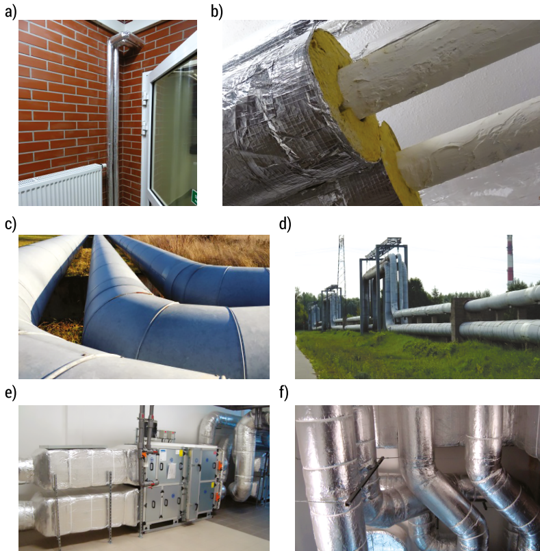
FIG. 7.5. Examples of thermal insulation made of mineral wool: a), b) fireproof thermal insulation of heating pipes made of mineral wool concentric pipes, protected by an outer coating of reinforced aluminum with high resistance to water vapour, c), d) mineral wool in a steel casing, e), f) mineral wool on the ventilation ducts (Source: photo by T. Teleszewski)
