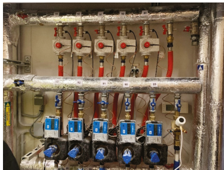
FIG. 2.23. Automatic balancing valves for distribution regulation (Source: Danfoss, 2022)
