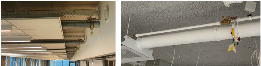
FIG. 2.15. Automatic balancing valves for cooling systems (Source: Danfoss, 2022)
