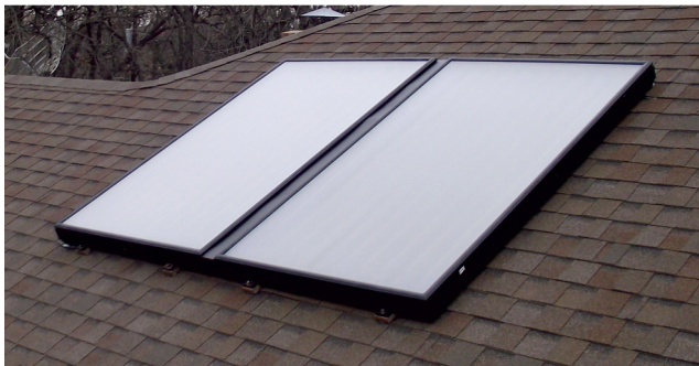
FIG. 1.20. Flat plate solar thermal collectors (Source: WEB-2)
