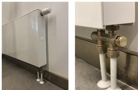
FIG. 2.21. Dynamic H type connection with integrated pressure regulator (Source: Danfoss, 2022)
