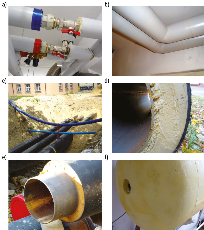
FIG. 7.1. Examples of thermal insulation made of foamed polyurethane: a), b) foamed polyurethane in a PVC housing, c), d), e) polyurethane foam with a casing pipe made of polyethylene of high density (PEHD), f) foamed polyurethane on the heat storage tank (Source: photo by T. Teleszewski)
