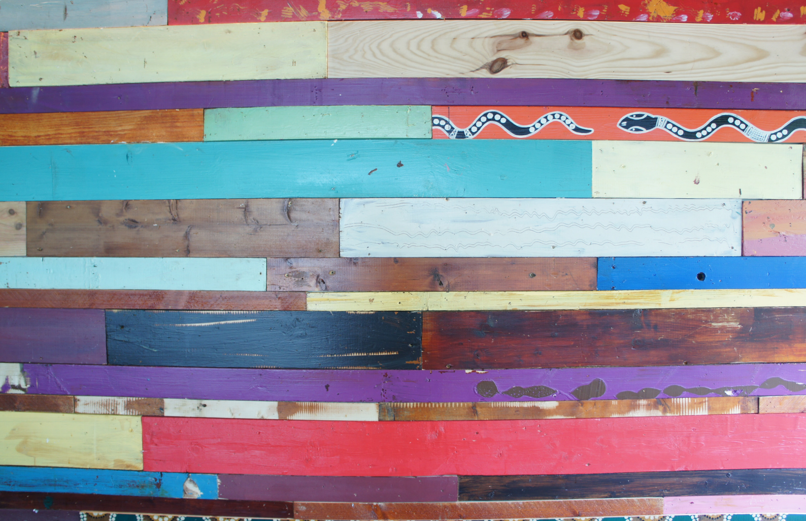
Fig. 2. Wooden panels reclaimed from demolished buildings and incorporated as wallcovering in a new location. Restaurant and music club situated in the complex La Cité de la Mode et du Design, Paris, proj. D. Jakob, B. MacFarlane; photo by the author, 2017
