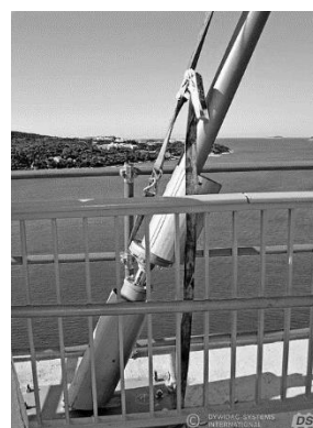
Fig. 5. Cable vibration dampers based on MR fluid technology ( https://www.dywidag-systems.com/emea/projects/project-details/article/dr-franjo-tudjmann-bridge-dubrovnik-croatia.html )
