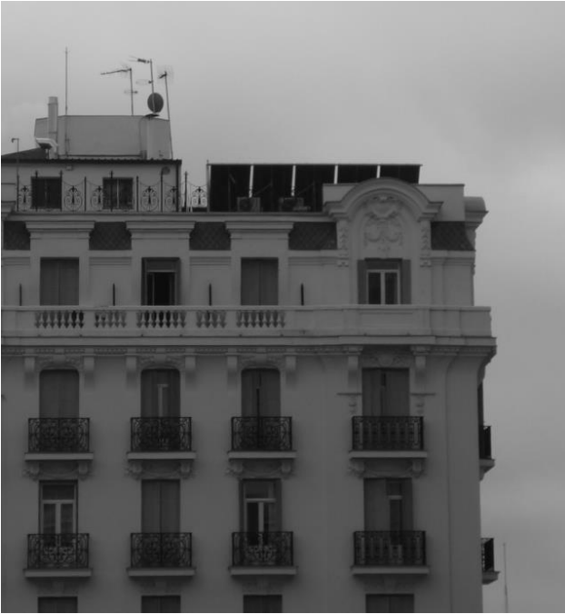
Fig. 3. The front façade of the hotel (photo D.A. Krawczyk).
